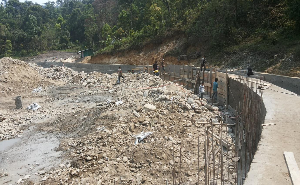
Construction of Boating Lake (Work in Progress)
